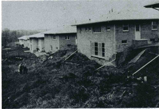
When acting force exceeds friction, real estate values perceptibly slide -- hence the term "Skid Row". Part of this slide in Des Moines was subsequently stabilized with lime. Watch for details in ASCE "Civil Engineering".
