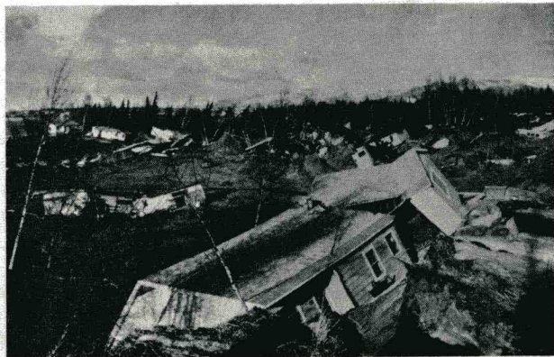
The March, 1964 Alaska earthquake densified lenses of loose sand, increasing pore pressure to cause liquefaction and trigger landslides. Clays also lost strength, helping the slides move along. This one moved laterally about 500 feet. For details see ASCE Jour. Vol. 93 SM4, July 1967. Photo courtesy Dr. H. B. Seed, Univ. of Calif.
