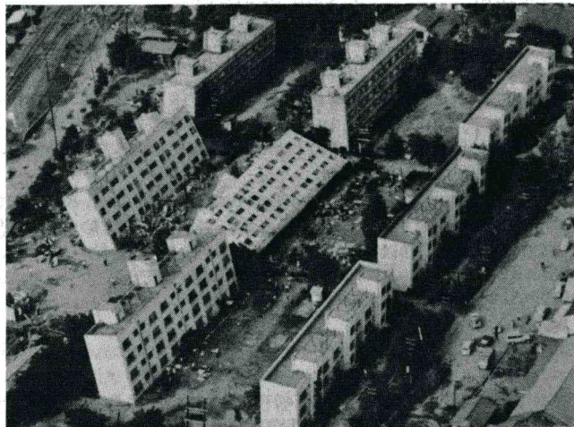
TILT! Aftermath of an earthquake which rumbled through Niigata, Japan, in June 1964. Vibrations reduced shear strength of the loose underlying sands, causing quicksand "boils" (right), plus extensive settlements and shear failures. For details see ASCE Jour. Vol. 93 SM3, May 1967. Photos courtesy W. G. Holtz, U. S. Bur. Recl.
