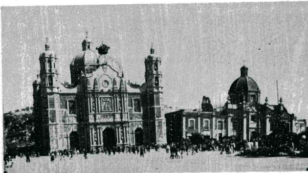
The Basilica of Guadalupe and the neighboring priests' home tilt in opposite directions. A buried rock ridge extends between them from the volcanic neck in back. The clay is thinner over the buried ridge, giving less total consolidation. The left corner of the Basilica is about 6 feet lower than the right.
