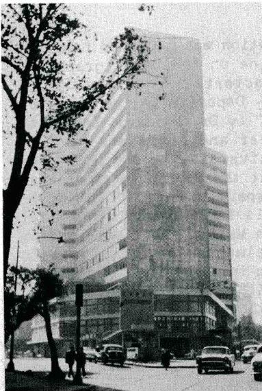
The Condominio Insurgentes office building is an example of a floating cell-type foundation utilizing water ballast. Provision is made to use additional atmospheric pressure loading if needed.
