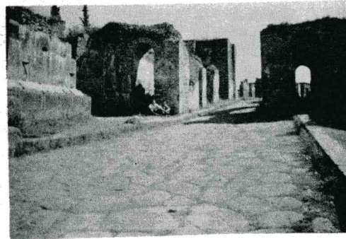
Pompeii street paved with slabs of lava. Street was preserved under hot ashes from Vesuvius in A.D. 79; note how tops of buildings are weathered and long gone.
