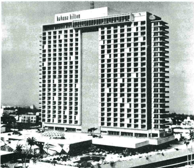
Habana Castro is firmly founded on capitalistic grout. Coral underneath the block-long hotel took 5500 cu yd of grout. (See inset at right.)
