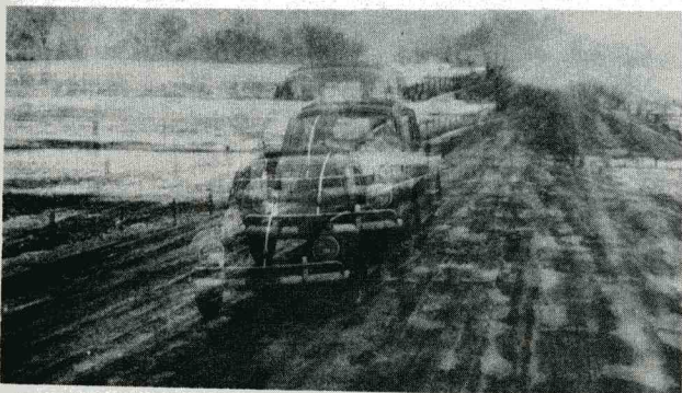
Frost heave raises some dynamic problems on roads, contributing to spring break-up (illustrated).
