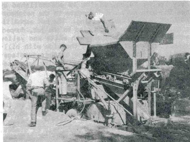
From such variegated heaps great asphalt roads grow. This central mix plant is adapted to use foamed asphalt, p. 3.
