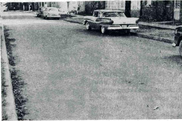
But another campus drive cheaply built with foamed asphalt. "Before" photos are on pp. 3 and 5 (under the machine). Engineering Experiment Station buildings are on the right.
