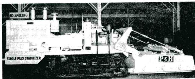
P & H Single Pass Soil Stabilizer decked out for application of foamed asphalt.
