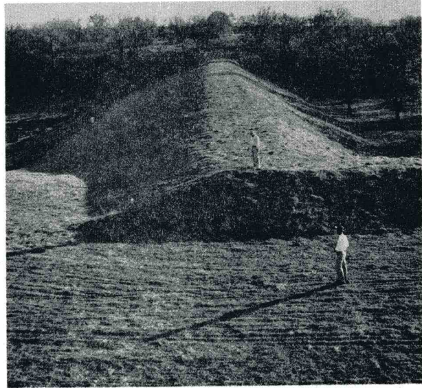
Typical small flood control dam, Snipe Creek Watershed, Kansas. Riser for the pipe outlet is housed by a protective screen at left center near the fence. In the foreground is the grassed emergency spillway.
