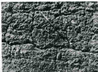
During initial drying or cure, calcium chloride roads shrink and gain density. Obviously something's got to give. Pencil for scale.
