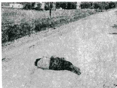
Engineer tests road-bed, finds it soft and rough. Looks like a good prospect for chlorides. Naturally, we had to go outside the state for this photo, Iowa roads being smooth as a lover's sigh. This road was later stabilized with salt.
