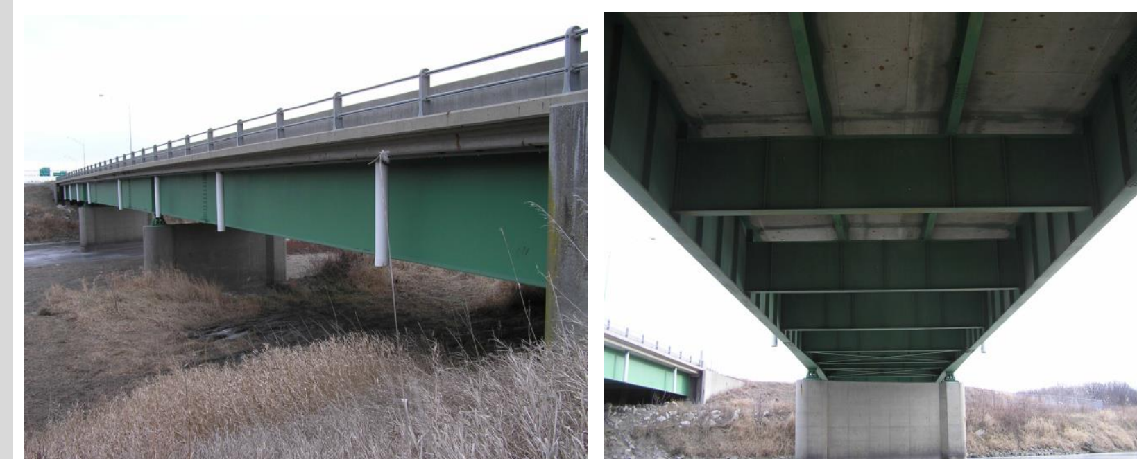
Fig. 2. Side and Bottom View of the US30 South Skunk Bridge (Lu 2008)
