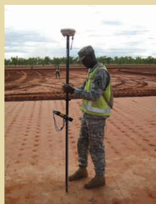
A military soldier uses a GPS device to help mark the runway.
