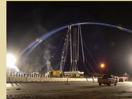
The above pictures show precast elements being placed on a bridge on I-235 in Des Moines, Iowa. The elements are used in accelerated bridge construction and are part of what's being studied by CCEE structural and construction engineers researching rapid bridge renewal.
